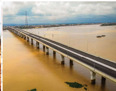
Figure 6: Construction Second Niger Bridge
