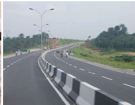
Figure 4: Construction of Keffi-Markudi road
