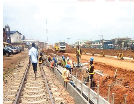
Figure 5: Lagos-Ibadan Rail Project Under Construction
